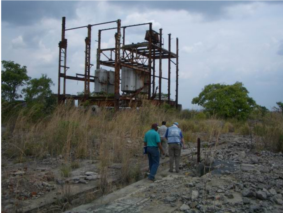
Figure 1: Remnant infrastructure at the former mill area (photo: Rene Nijenhuis, Joint UNEP/OCHA Environment Unit)
