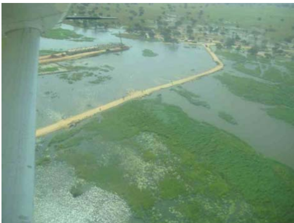
Warnock Bridge from East side – Finne Lucey 30-10-08
