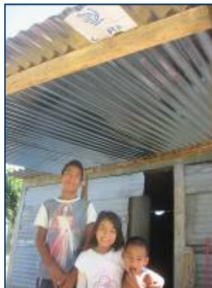
Zinc sheets and wooden boards after installation © IOM
