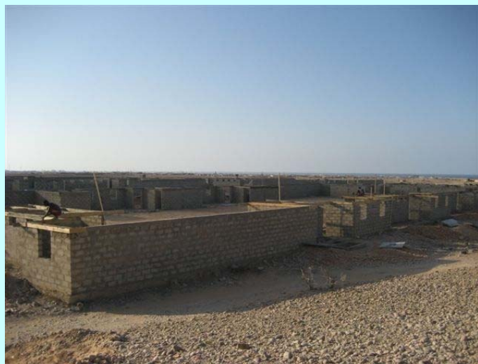
Permanent shelters for IDPs/urban poor under construction in Bossaso. Source: DRC
